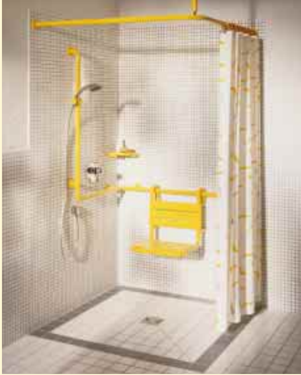
Universal design makes this washroom barrier-free and accessible for all users.
